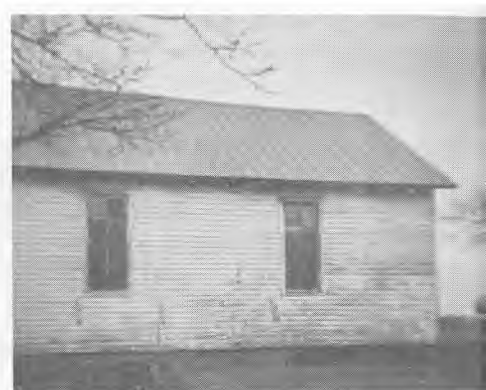
Frame Kishwaukee School On Farm on Rothwell Road
