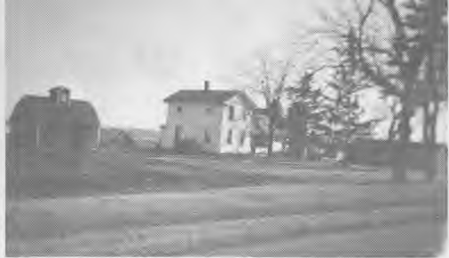
First Rothwell Farm on Stillman Valley Road Part of Underground Railroad
