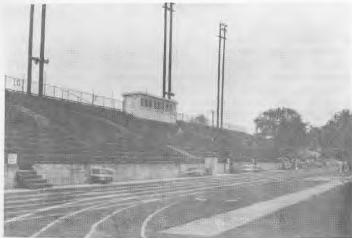
Grandstand at Beyer Stadium
