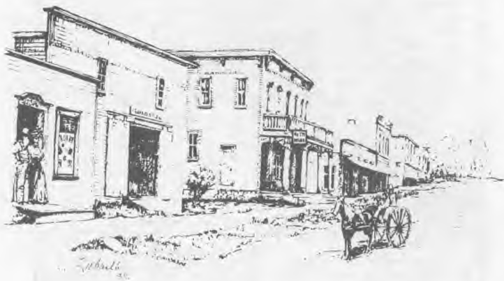
150 S. COURTLAND STREET - Looking East to Main Street
