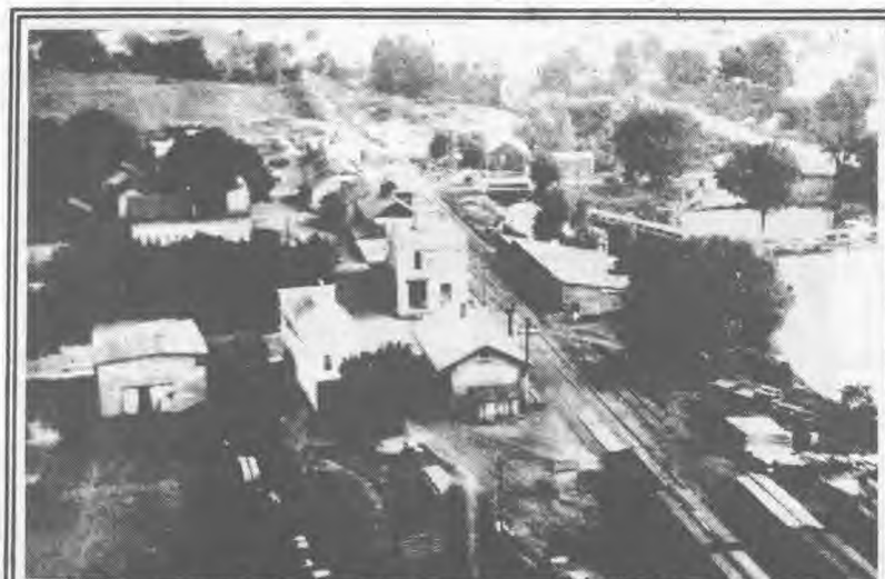
In 1912, when this photograph was taken, Squires Street was an alley that ran along the railroad tracks. Pictured from bottom to top are the railroad depot, now the Melting Pot; the mill, now the Old Mill Restaurant; the granary and bean plant, now Buckley's Mall. The building to the left of the depot was once part of the Squires bean processing operation, and today houses the Weaver Shop.
